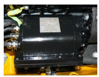
All circuits and components are located in a flameproof enclosure.
